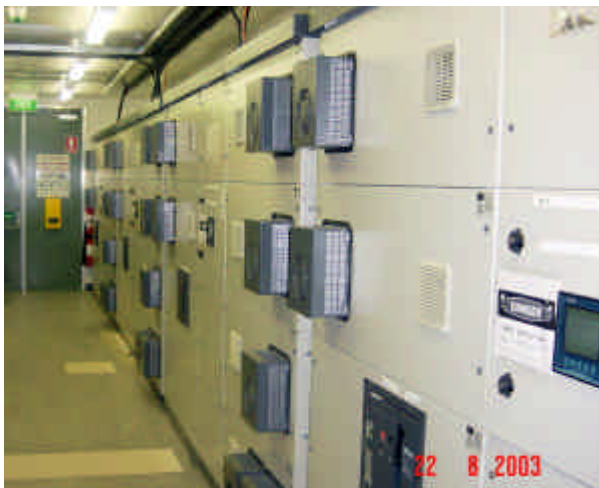
Figure 1: Challicum Hills' Elspec Equalizers
