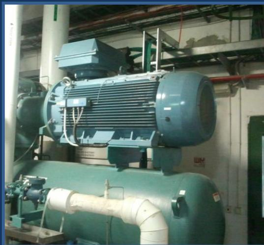
Figure 1a: 700 HP, 400V/50 Hz Cooling Compressor - Carlsberg
