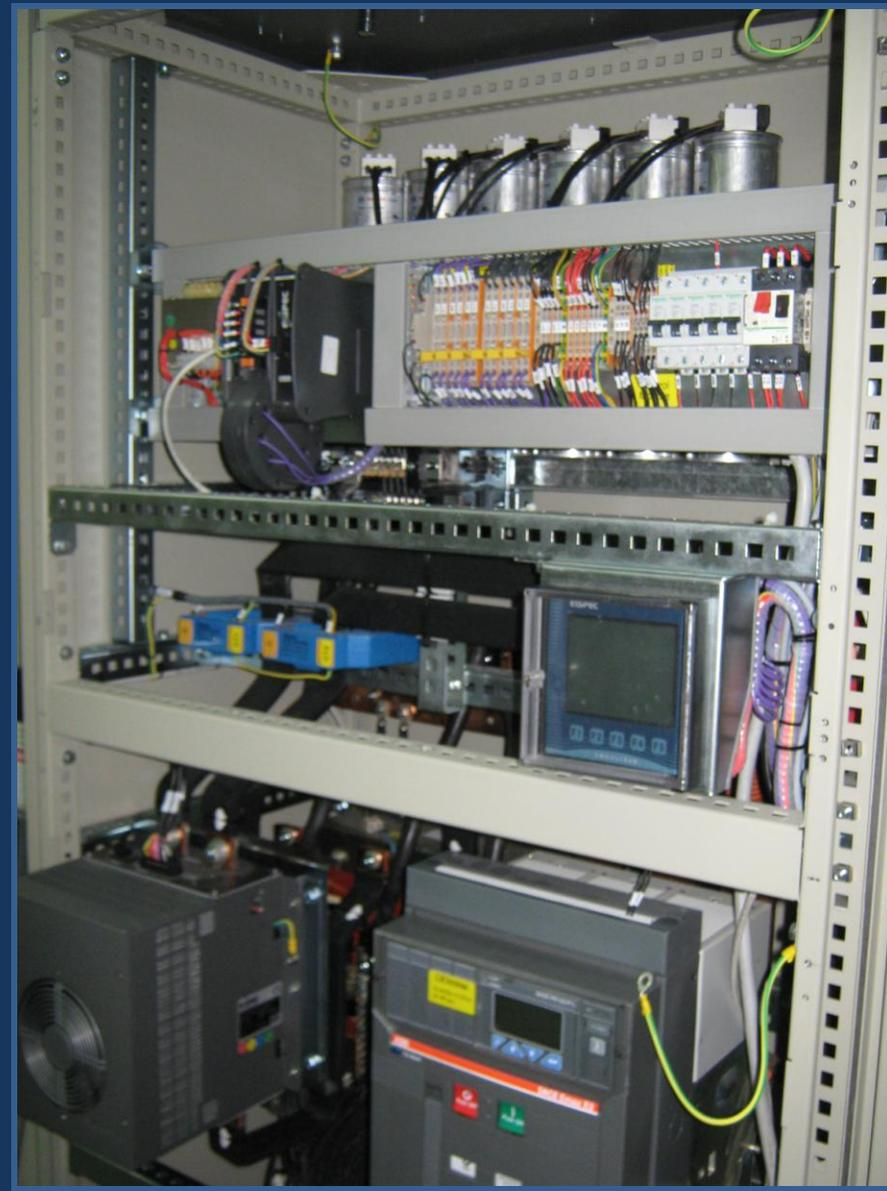
*Figure 1c & d: EQ-ST & EQ Compensation Systems, Including G4K BLACKBOX PQ Analyzer & Controller*
